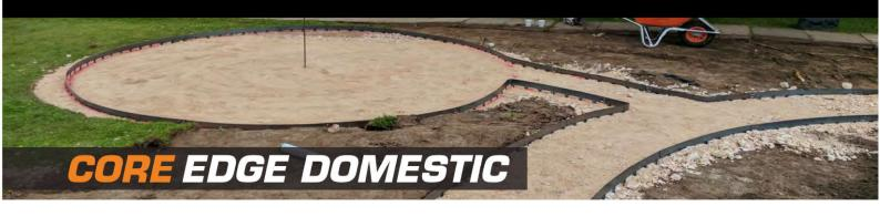
The CORE Edge domestic range is manufactured from 1.6mm mild steel and is hardy enough to handle ride on mowers and light vehicles. This flexible steel edging can be quickly installed with no specialist tools required. Easily Forming both straight lines and curved radius, or bent on site to form precise angles. It provides the perfect edge restraint in a variety of landscaping applications.
