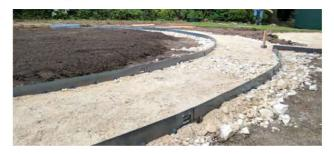
All of our edgings except our weathered steel (Cor-Ten effect) have a 20-micron Galvanised Zinc coating. Our (RAL) coloured edgings have a further 110-micron UV resistant polyester powder coating preventing colour fade, forming a durable scratch resistant barrier guaranteeing a 20yr plus product life.
