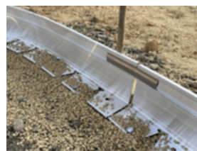
Step 3: Joining and Expansion of Lengths
